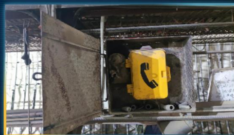
防爆电话安装示意
